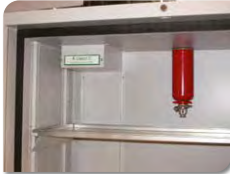
Fire-extinguisher installed in a safety cabinet
